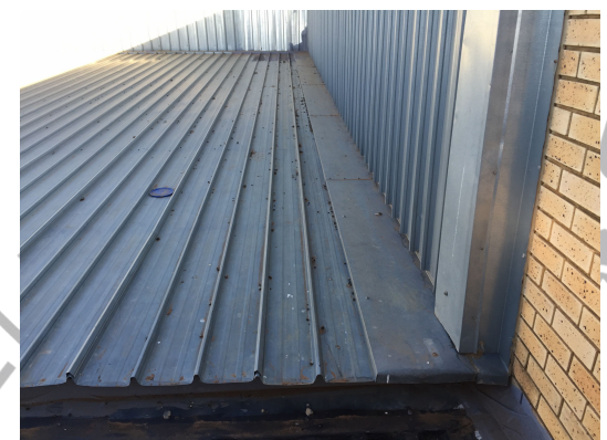
Metal sidewall flashing with vertical cladding
